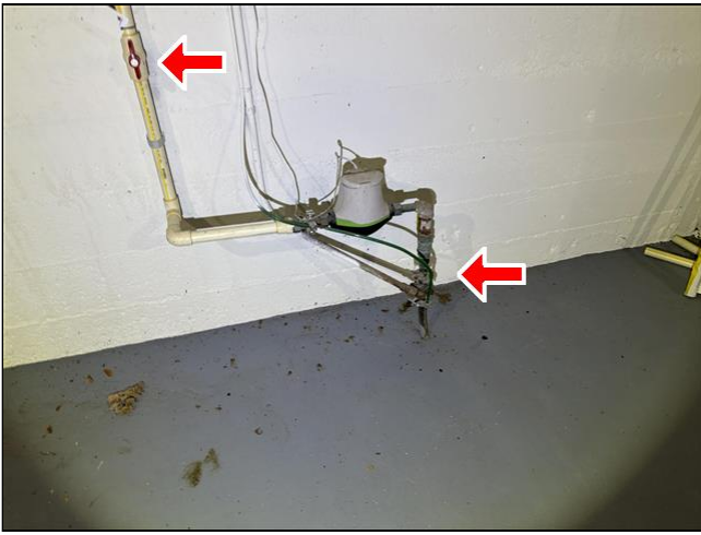
6.3 Main water shut off for home is located in basement left of the water softener.
